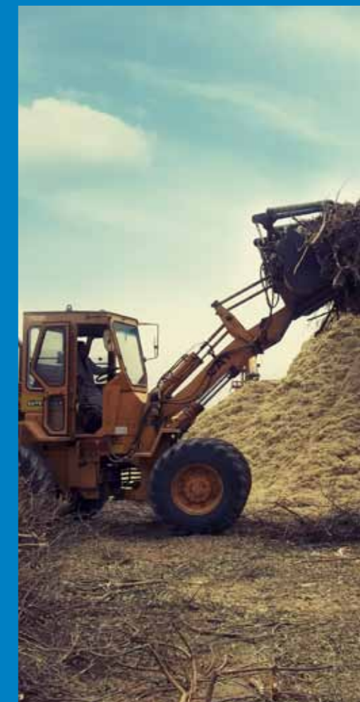
Tawazoon provides biomass and RDF as alternative fuels to heavy energy consumers such as cement factories
